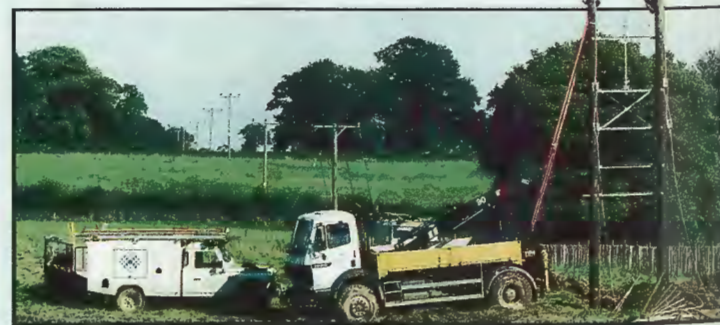
Reinforcement work means that the power network is more able to withstand winter weather.
